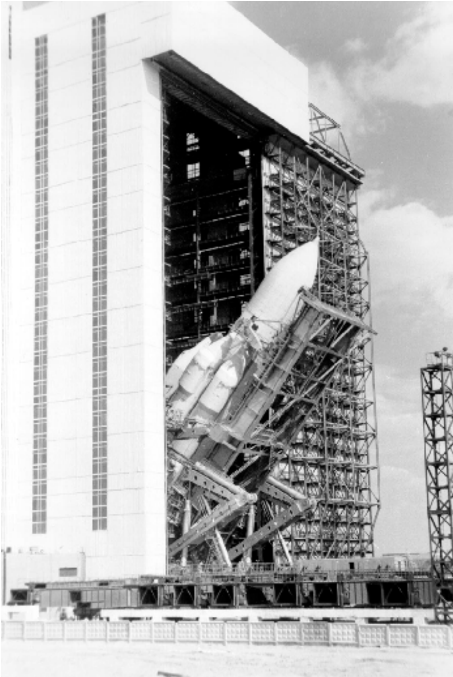
Energiya being erected inside the Dynamic Test Stand ( source: www.buran.ru ).
