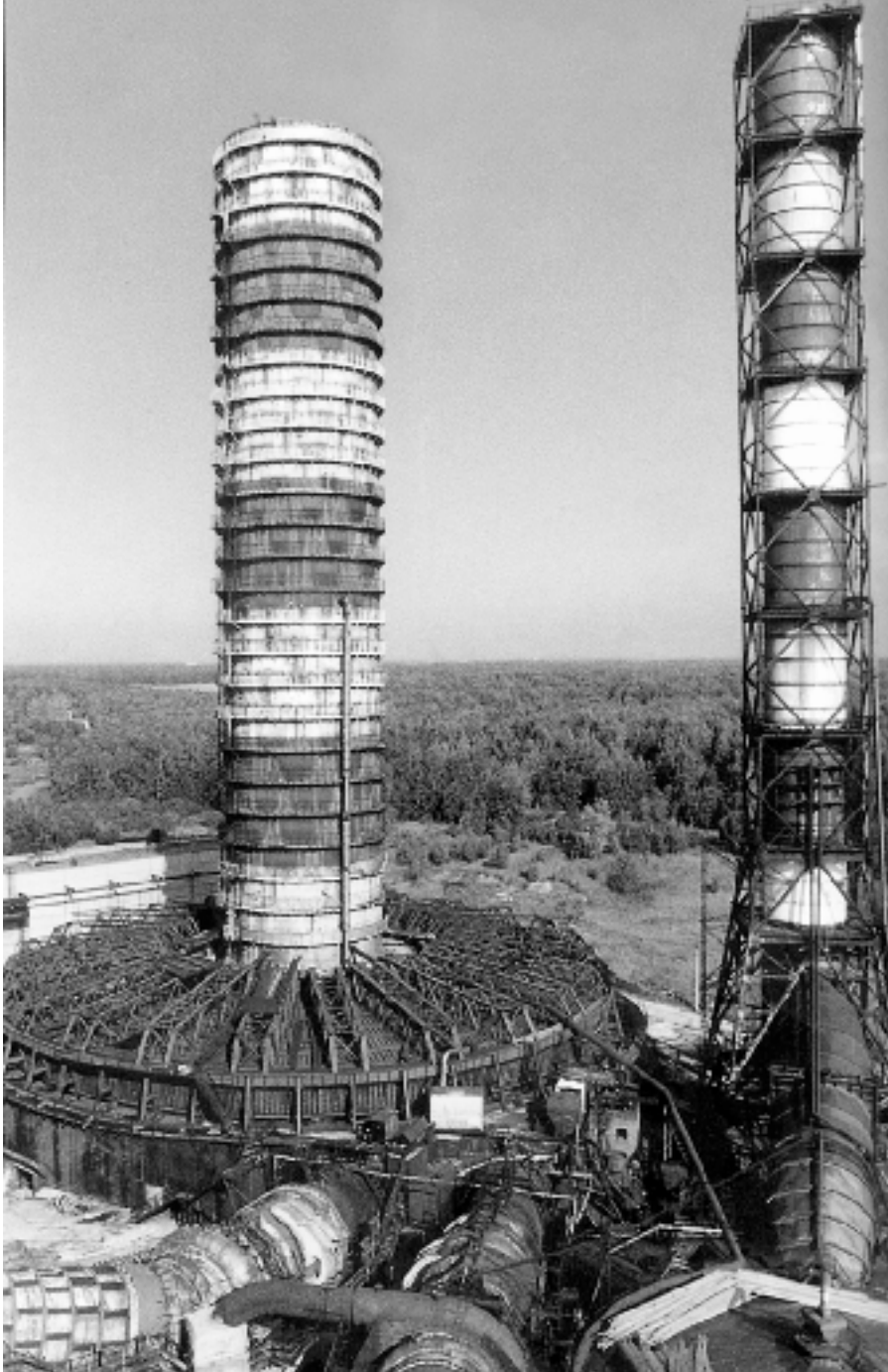
Energomash engine test-firing stand ( source : NPO Energomash).
