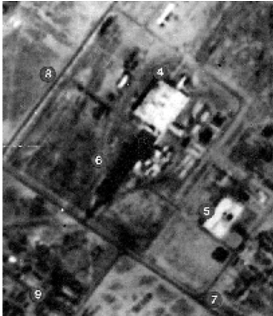
SPOT images of Baykonur runway (top) and assembly buildings. MIK RN and MIK OK are in positions 4 and 5 ( source: SPOT Image ).
